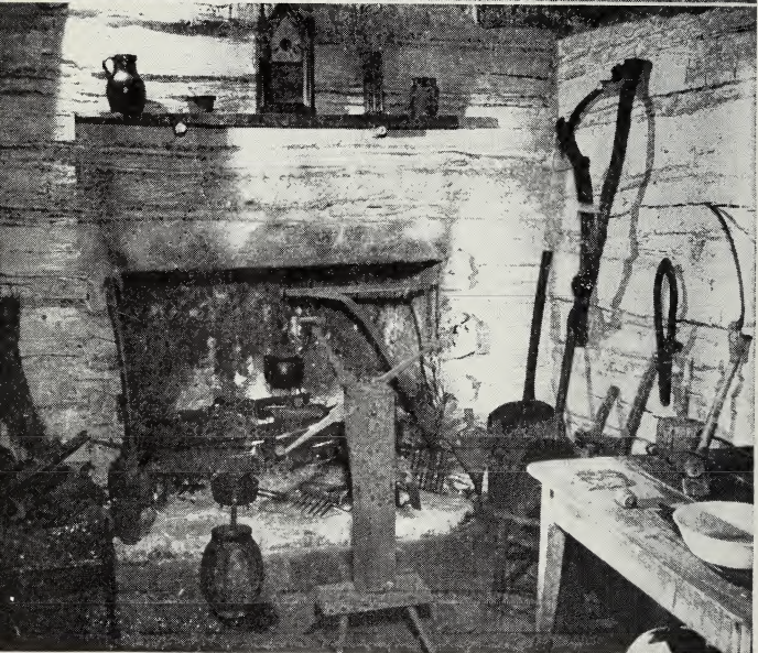
THE BIRTHDAY CABIN from the outside and inside. The reconstructed interior of the Chicago Historical Society views the room from the bed where Lincoln was born.
